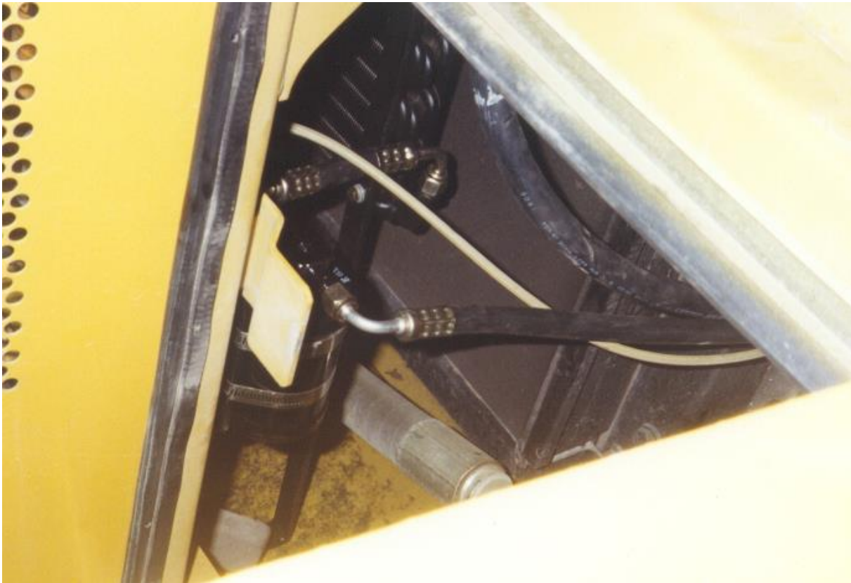
Drier in location with hose from condenser.
